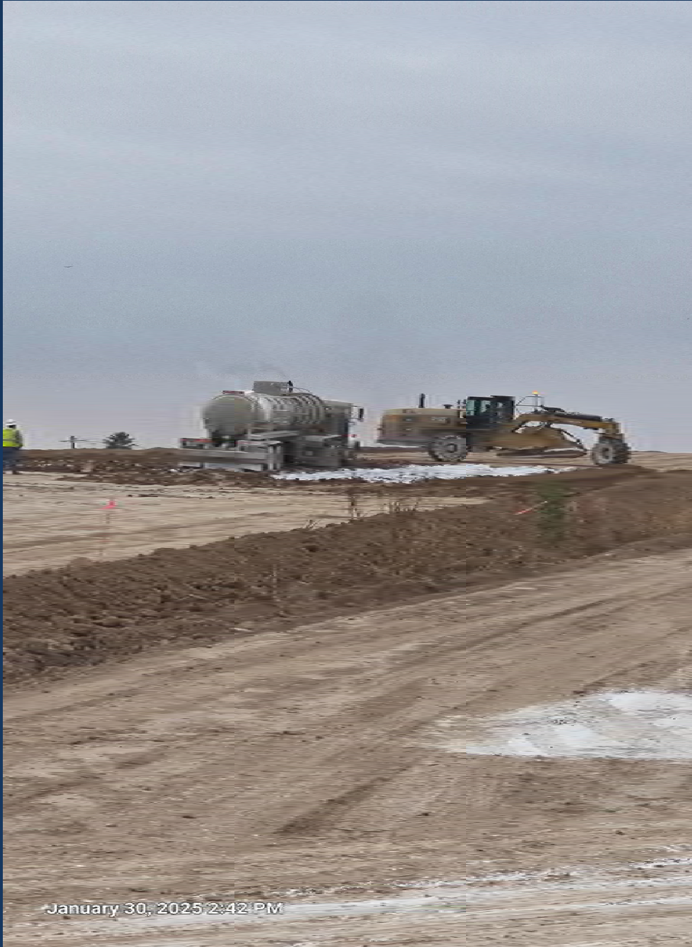
Lime placement in base at Jackson (FM2061)
